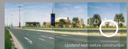
Upstand kerb before construction
