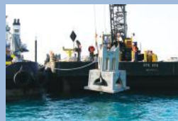
Our contribution included the supply of over sixty precast wind towers and anti-trawl devices which will be used in improving fish stocks around Bahrain.
